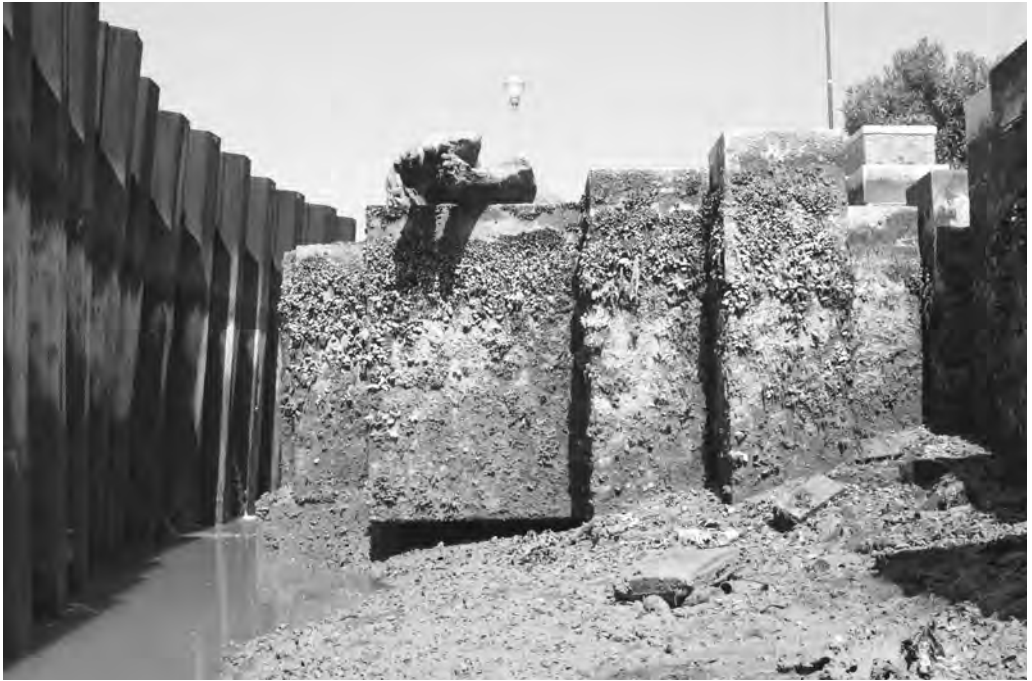
7. Monument to the Partisan Woman , view of submerged stone exposed during restoration. Photograph courtesy the Office for the Protection of Architectural, Natural, Historic, Artistic, and Ethno-Anthropological Heritages in Venice and Its Lagoon, Comune di Venezia.
